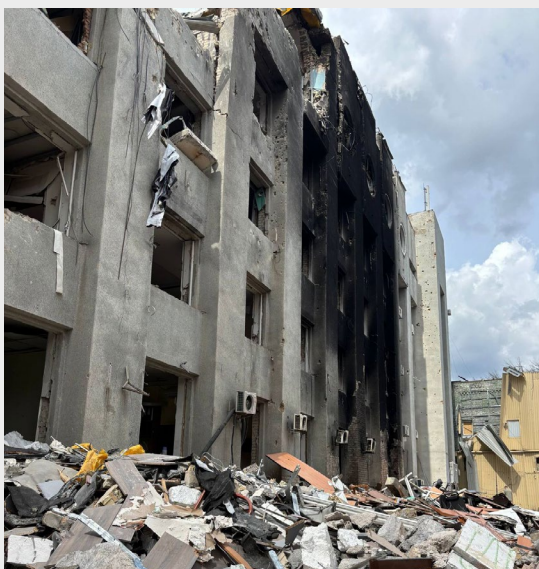
The building of the Main Directorate of the SES in Kyiv Oblast, damaged in the aftermath of a Russian attack on Kyiv on 24 May 2026. Photo: 24 Channel. 10
